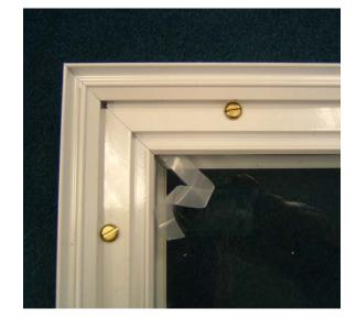
4. Once the panel has been stuck to all four glazing beads turn the assembly over and insert the wedge gasket between the glass and the top surface of the aluminium frame. Make sure that the mitred corners of the gasket are pressed into each other.
